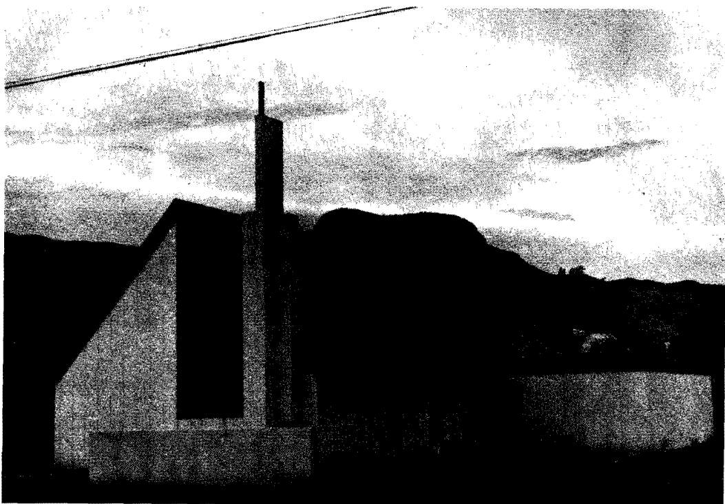
The new Methodist Church, dedicated February 7, 1965. Courtesy of Floyd McDaniel
